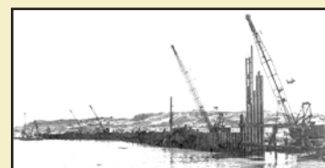
Figure 3 Pile drivers work to complete first berth, Naha, Okinawa
